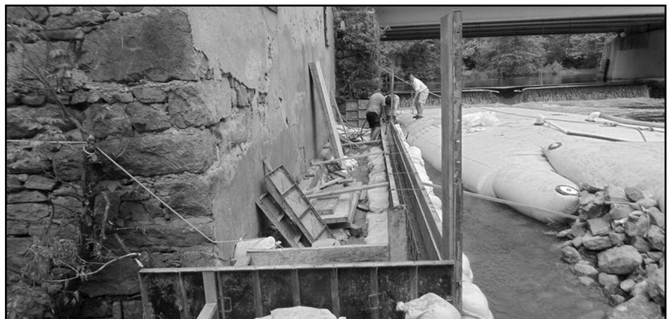
*Pouring concrete slab for reconstruction of the tailrace island*
