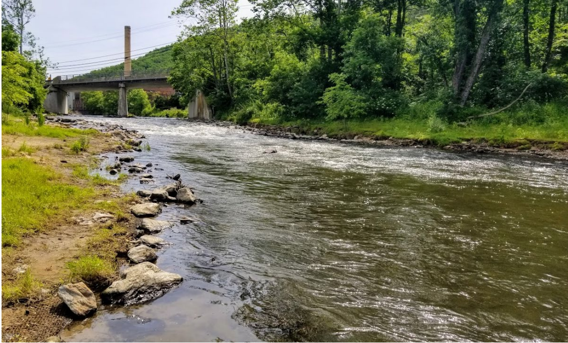
Image of the site after restoration. This is an upstream view towards State Road 519 from taken from the dam former location.
