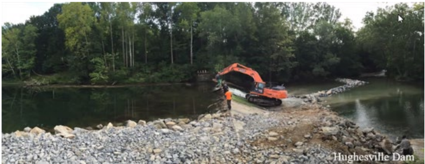
Image of the Hughesville dam being notched in 2016.
