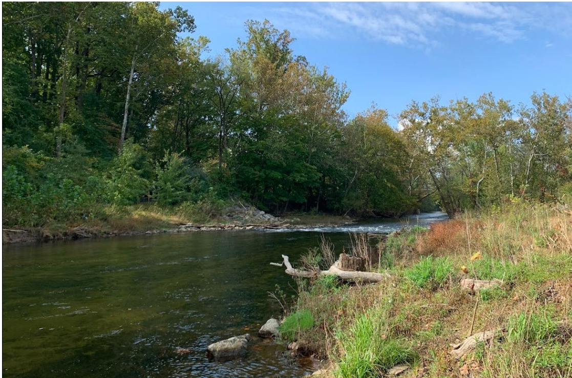
Image of the site after restoration. This is a downstream view towards where the dam structure was located, from the location of the former impoundment.
